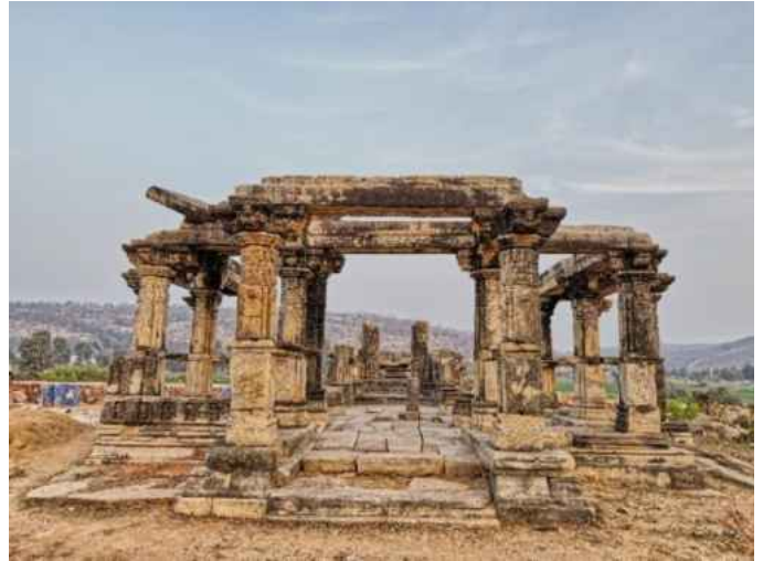
A ground view of Kotan ki Deori No.1
